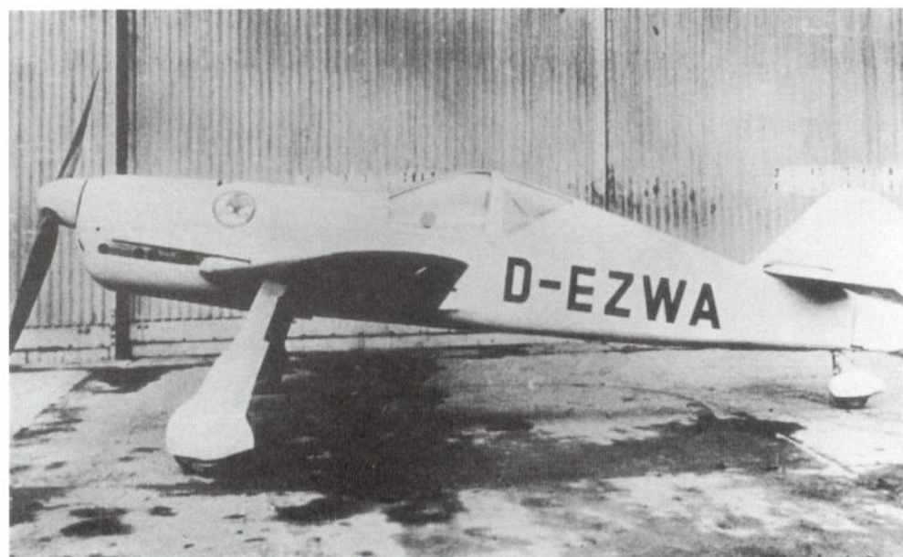
55: Almost a Luftwaffe fighter-trainer, D-EZWA was the prototype Skoda-Kauba V4 which was designed by a team led by Austrian Otto Kauba, based at Cakowitz, near Prague, in 1942. Trials with four improved further prototypes led to the type being ordered into production as a potential standard Luftwaffe trainer aircraft. The whole idea was effectively sabotaged when the first five Czech-built production aircraft were found to be so badly constructed that the whole project was abandoned
