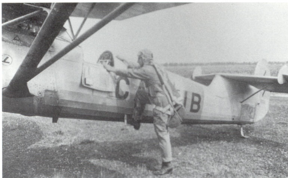
53: Excellent closeup of student pilot Reum as he climbs aboard Focke-Wulf Fw 56, CA+IB, for a high altitude flight to 4000 m. The overall grey finish shows numerous details, including the yellow fuselage band, the Focke-Wulf company logo just above the strut root, details of the hinged access hatch and the data table below the tailplane. This identifies the machine as belonging to LKS 2 based at Berlin-Gatow, although actual flying took place from Güterfelde and Reinsdorf (AMC)
